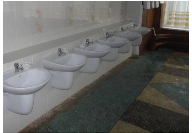
Picture#24: Typical required wall supported sink with automatic faucets for cold water
