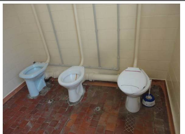
Picture#33: Condition of existing bathrooms
