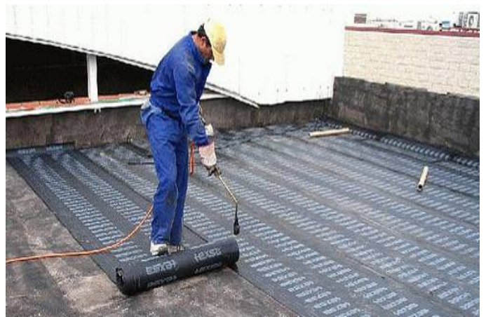
Picture#08: Typical roofing work
