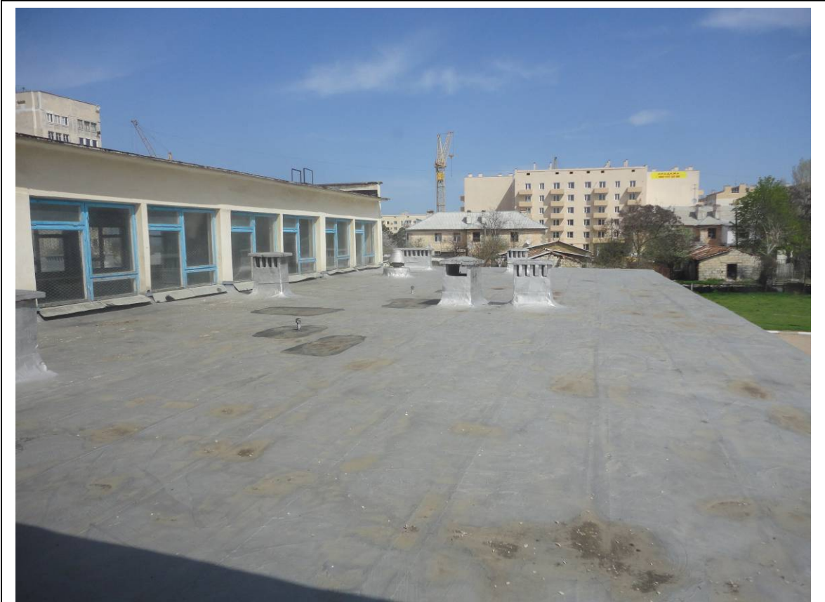
Picture#11: Roofing area to be repaired.
