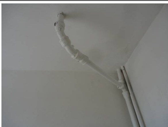
Picture#32: Typical drainage piping from floor above to be replaced with new PVC piping and covered under drop ceiling and new wall surfaces. No piping to be seen in bathrooms after renovation is complete.
