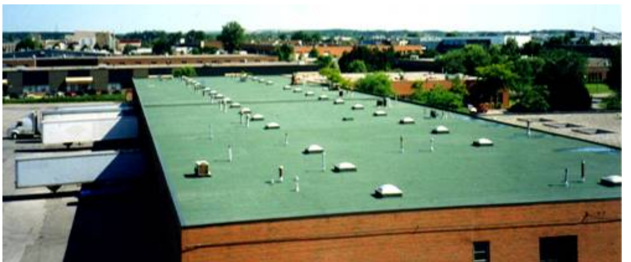
Picture#09: Typical required finish
