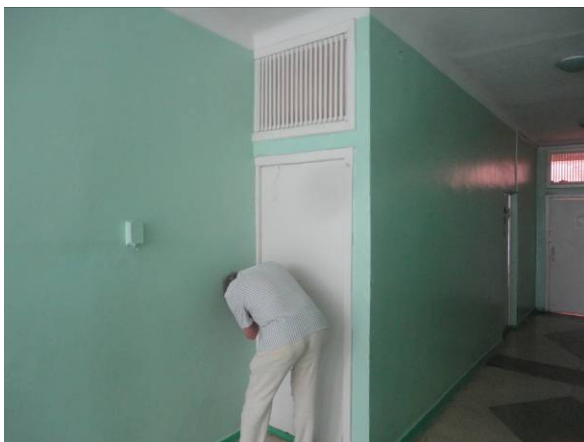
Picture#36: Replace door and louver for ventilation over the doors of the 6 bathrooms in West Wing
