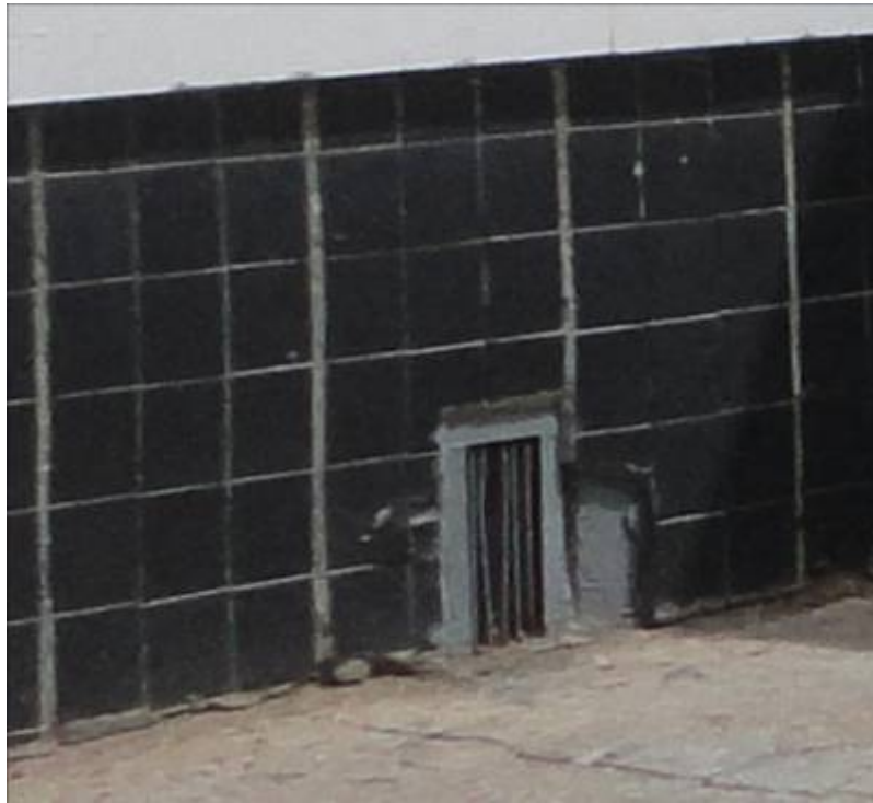
Picture#116: Typical ventilation window or opening for basement
