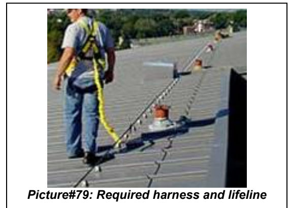
Picture#76: Required harness and lifelines
