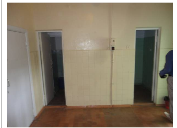
Picture#65: Interior of locker rooms
