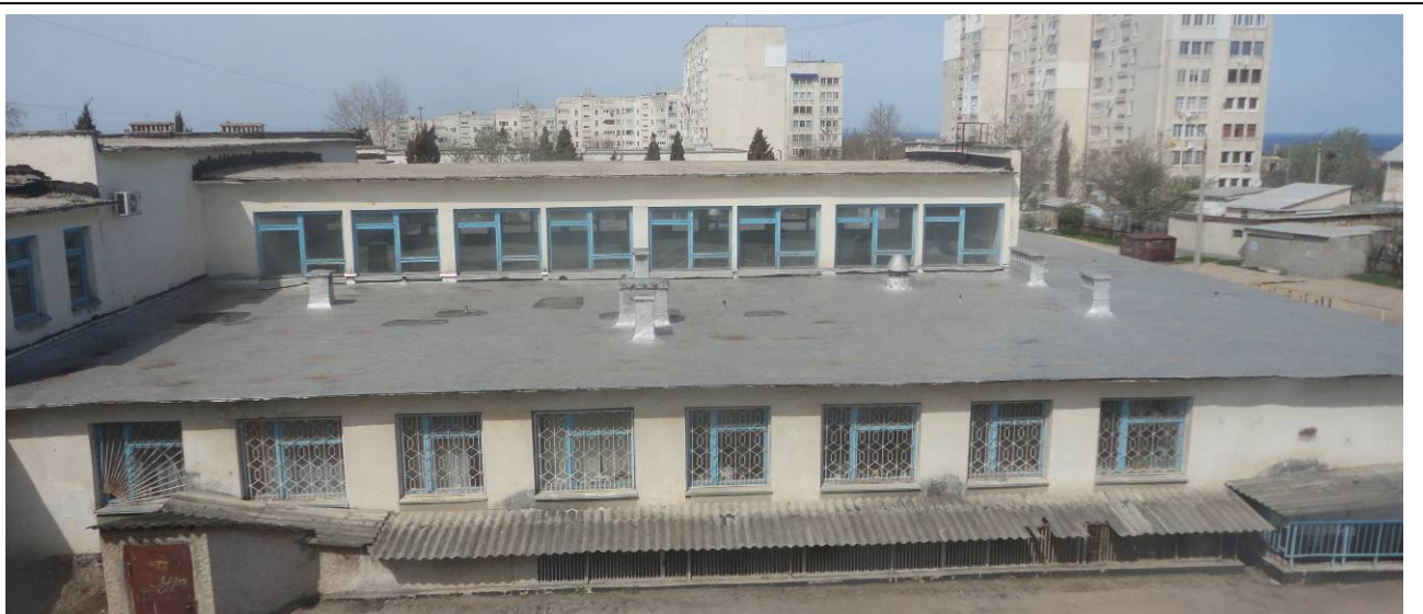
Picture#10: Roofing area to be repaired
