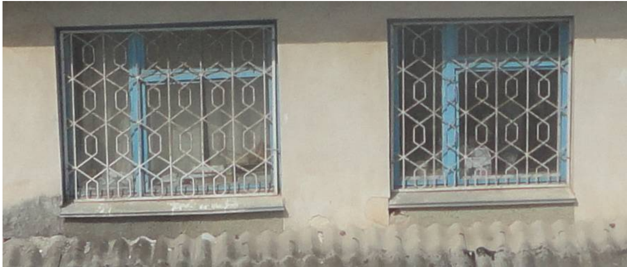
Picture#115: Typical security bars for windiws included in Option-3
