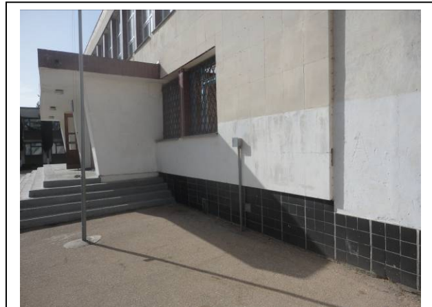
Picture#100: All ceramic tiles to be removed.
